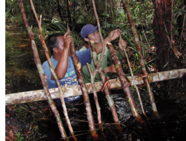
Using local material to dam small drainage canals in Sebangau National Park in central Kalimantan. These simple and thus cheap dams are effective in rewetting the peat areas upstream.
