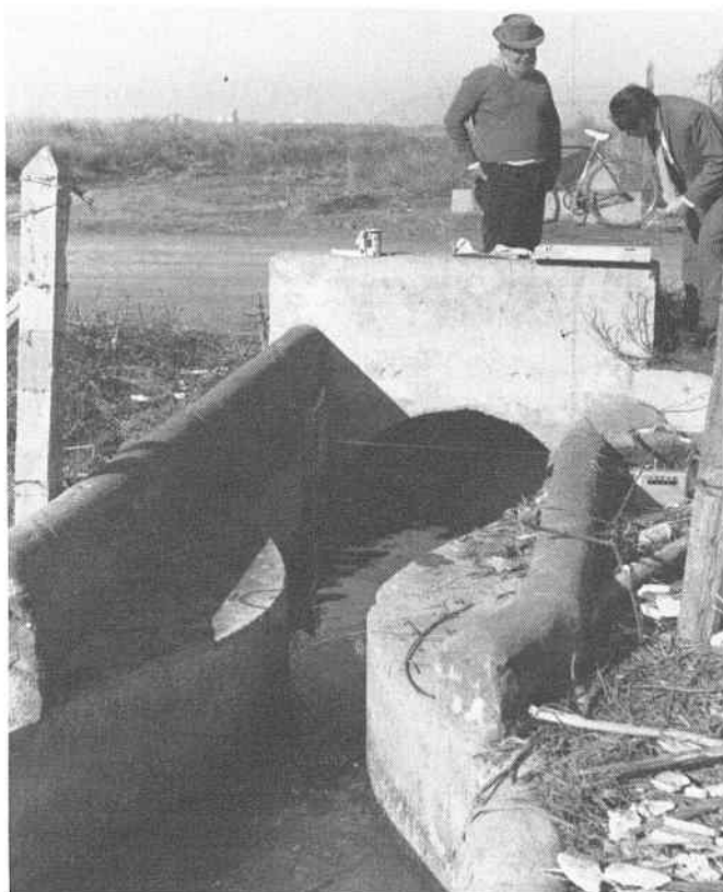
Photo 2 Throatless flume with rounded transition
